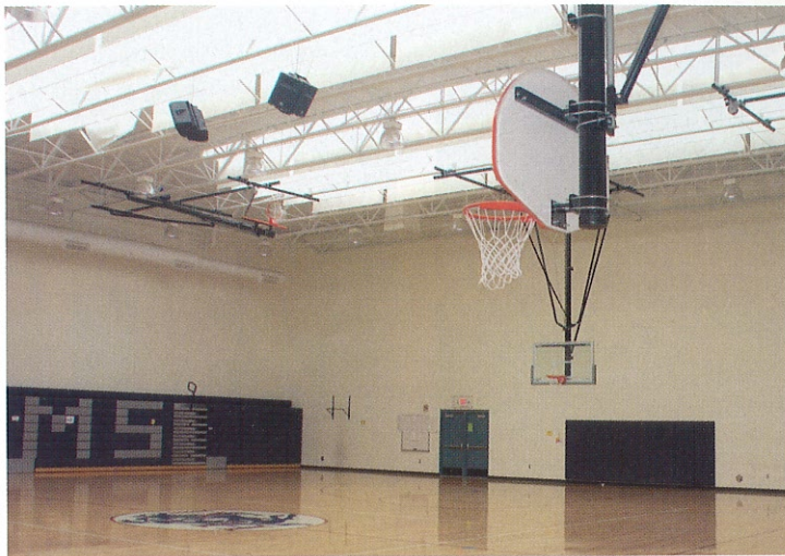
The architecture firm Innovative Design has used skylights in large rooms, such as this gymnasium at Heritage Middle School. Baffles block direct sunlight.
