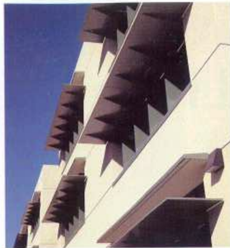
Light shelves bounce light through short windows onto classroom ceilings, and shade the glass below.
