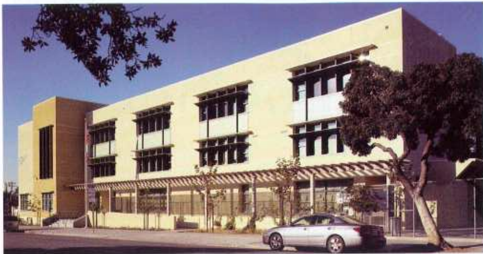
Harley Ellis Deveraux, an architecture and engineering firm, and Greenworks Studio, a sustainable design consultant, recently completed Charles H. McKim Elementary, a CHPS school in Los Angeles.
